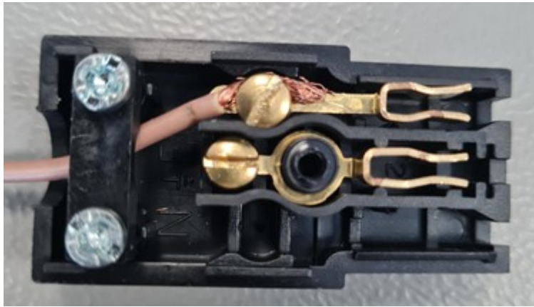
Figure 15-3. Wire Clamp Added to Hold Wires in Place
